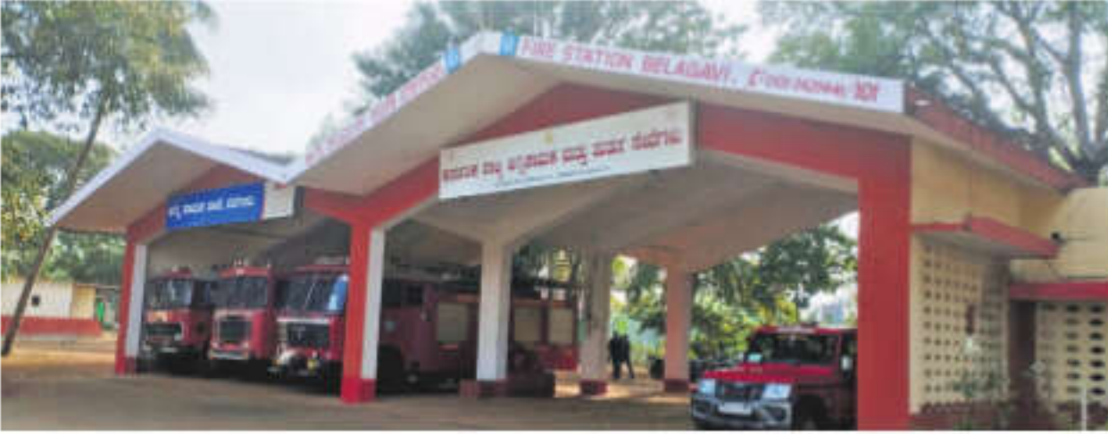
A view of the existing fire station | EXPRESS
