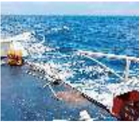
Damaged railings on the port side of BRP Datu Magat Salamat after a collision. AFP
