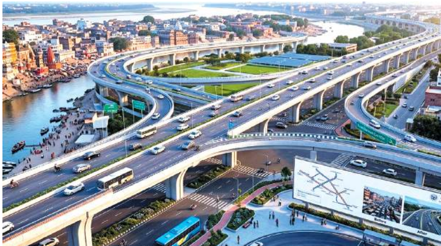
The Rs 10,998-crore, 43.218-km Varuna Elevated Corridor in Varanasi is set to transform the transport network by providing a high-capacity route between NH-31 and Varanasi.
